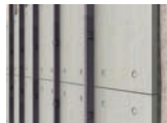
② 粘锚ZX外墙防火保温板
